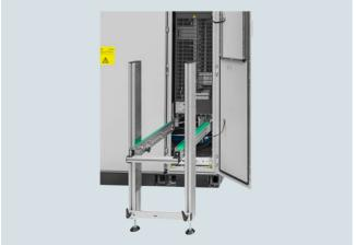
The mounting device is used to install or remove liquid-cooled power units (Line Modules, Motor Modules) in or out of a control cabinet. The mounting device can be used if the power units are mounted on mounting rails, which at the front have two M6 threads at a vertical distance of 20 mm to attach the mounting device.
