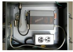
Wireless Ethernet Modem mounted within an enclosure located inside bunker
